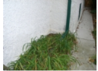
Picture Date:10/26/2006 Comments: This downspout in front on East side drains next to the house.
