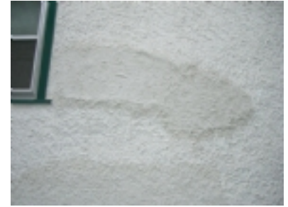
Picture Date:10/26/2006 Comments: Wall repair made to stucco.
