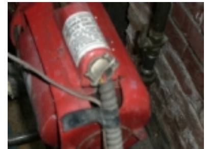
Picture Date:10/26/2006 Comments: BX connector needs to be reconnected.
