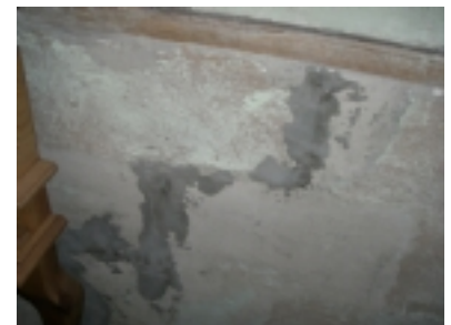
Picture Date:10/26/2006 Comments: Patching of cracks in basement foundation wall.
